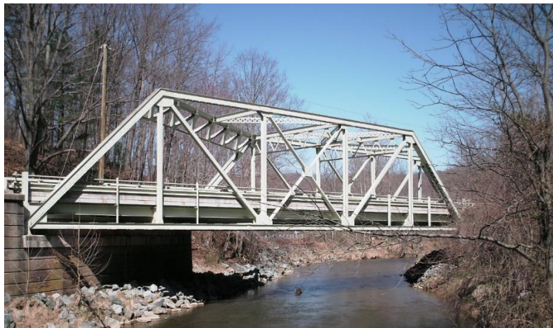
Figura 1.5.a. Rocks Steel Truss Bridge, Maryland, U.S.A.
