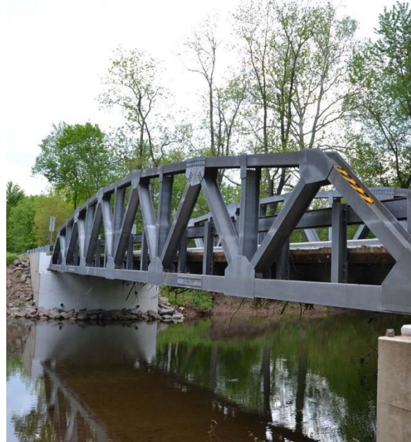
Figura 1.4. Tom's Creek Bridge, U.S.A.
