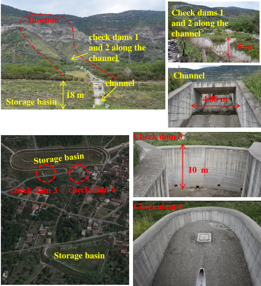
Figure 8.8 Overview of control works in Tuostolo basin.
