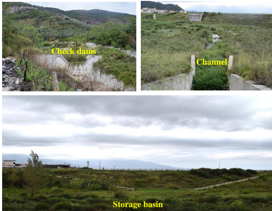
Figure 8.16 Check dams, channel and storage basin filled by vegetation (photo taken in September 2017).
